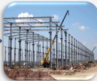
3-Install beams
