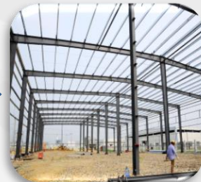
4-Install secondary steel
