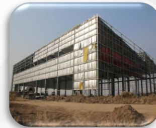
6-Install roof and wall panel
